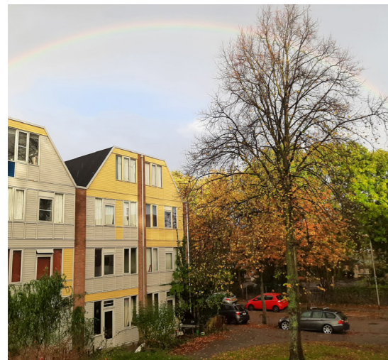
A picture containing tree, outdoor, sky, building
